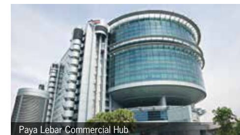
Paya Lebar Commercial Hub
