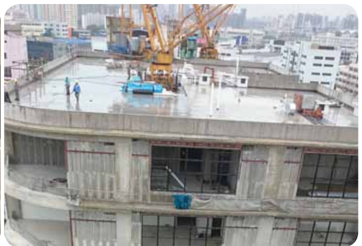
Construction at HH@Kallang
