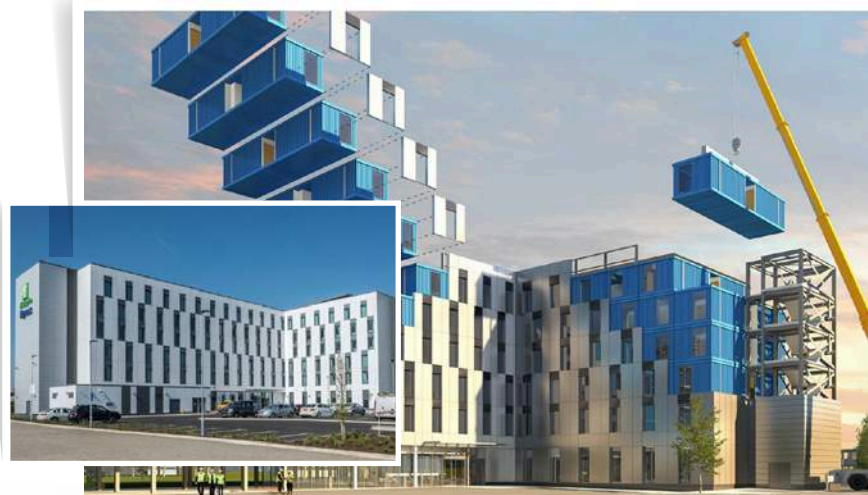
Holiday Inn Express modular hotel development at Trafford City, Manchester
